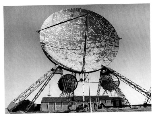
Tropospheric scatter dish, NATO Forces Scatter Station, Stenigot, Lincolnshire. Built in 1960. Made obsolete by satellite communication, and shortly to be demolished RCHME Crown Copyright
